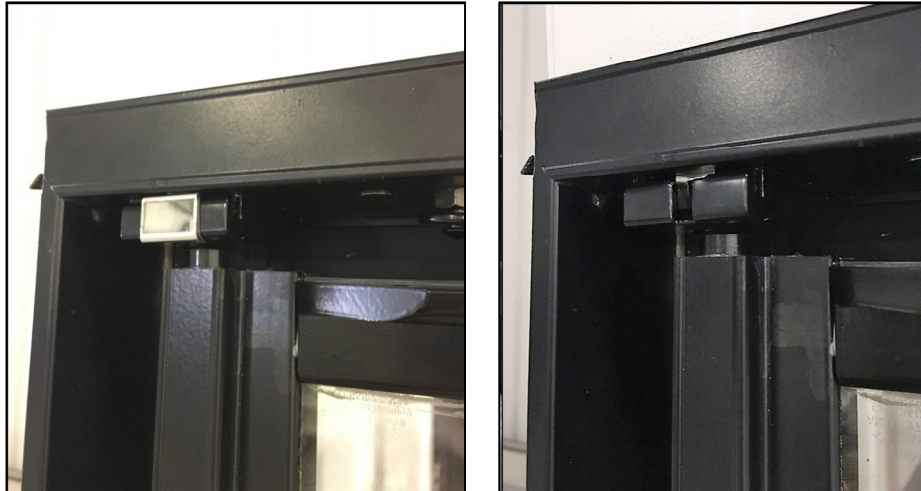
Figure 12 - 13. Unclip Hinge Pin Cap
